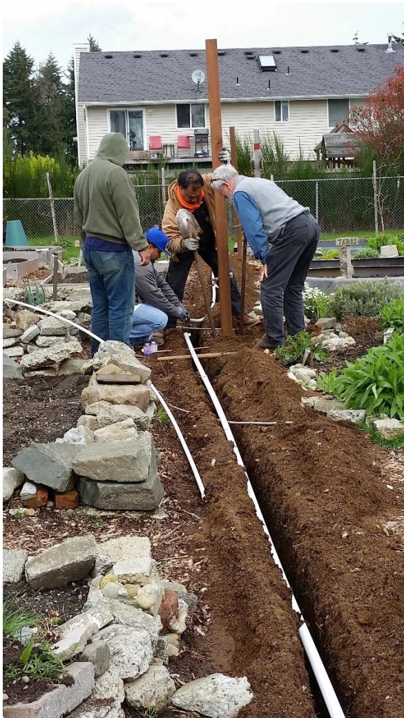
Irrigation System Being Installed
